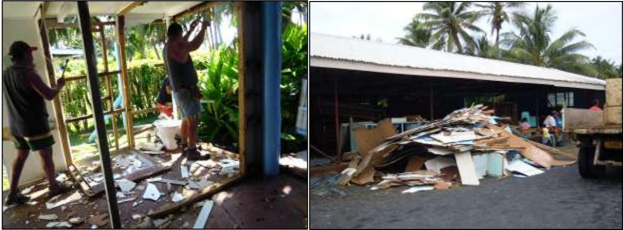
Men and boys at work; day 1 of dismantling the Matavera CICC Sunday School Hall before building a 2-storey replacement on the same spot.
