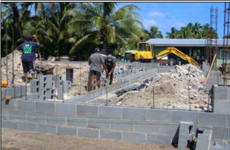
Saturday 20 September, brick-work is coming along just fine, and the structure is starting to take shape and look like a building.
