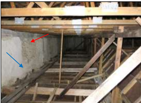
Figure 2: Existing ceiling void. Note the infilled windows from the lowering of the walls c.1944 (red, and redundant wall penetrations for (subsequently removed) original beams (blue). Source: Image by author, August 2014.
