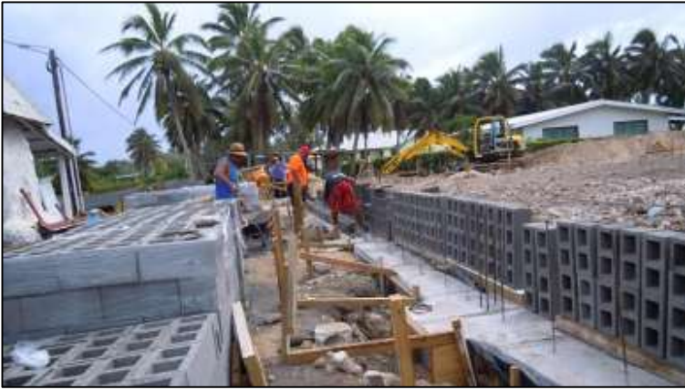
Saturday 13 September, foundation mortar is down and ready for the commencement of the brick-work.
