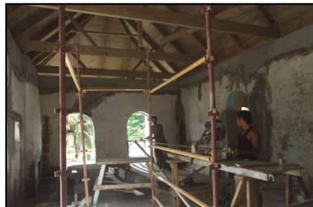
Work in progress, administration office, Takamoā
