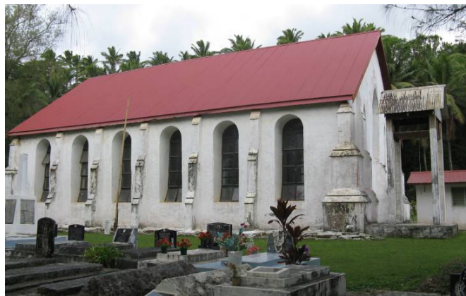
Above: the same building 117 years later. Notice the same number of windows and the 2 pillars on the front left and right corners. The first 2 photos were taken/reproduced from original photos provided by the Assistant Minister for Oneroa. All photos were taken by Tekura Potoru, CICC Director of Publication, November 2008.
